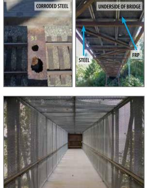
used for the ADA compliant walking surface of the bridge. The 12% open area of the grating allowed both water and sand to pass through. Fibergrate's FRP solutions provided the City of Everett an extremely low maintenance and cost-effective option for repair and will provide the visitors of Howarth Park years of safe access to this hidden beach treasure.
